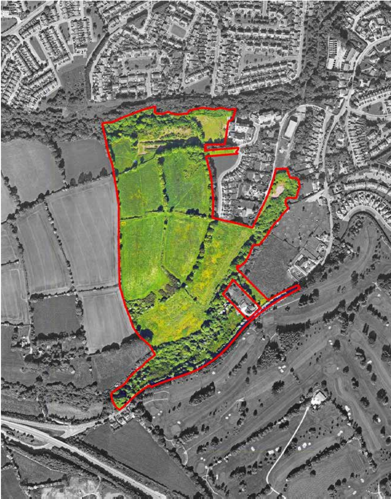
Figure 1.1: Aerial View of Proposed Residential Development Site
